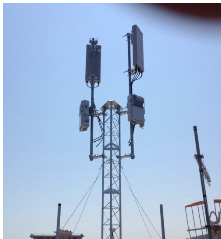
Exhibit 1: Tower with a GO base station
